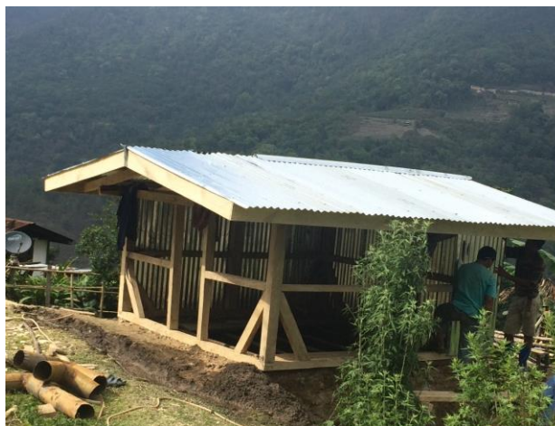
Pic: 5; Cardamom dryer installation at Dagana
